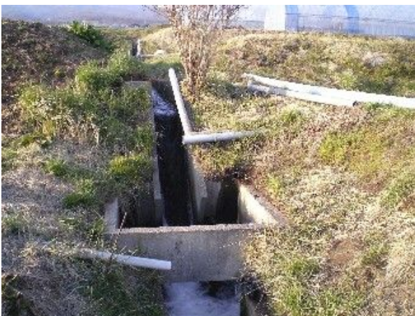
pic.3 before construction
