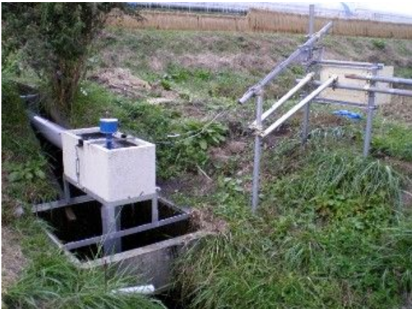
pic.4 after construction
