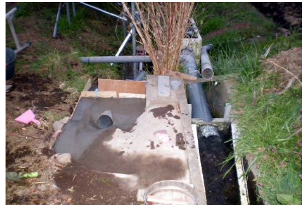
Pic.14 repair of embankment
