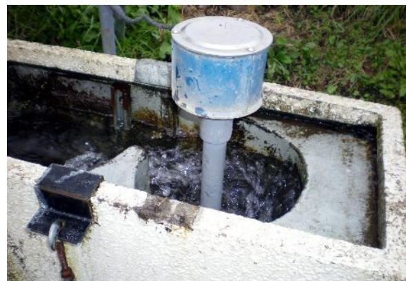
Pic.1 200W hydroelectric generator
