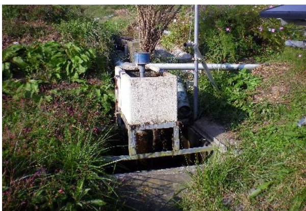
Pic.4 after construction
