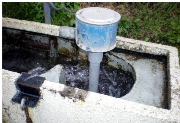
Pic.1 200W hydroelectric generator
